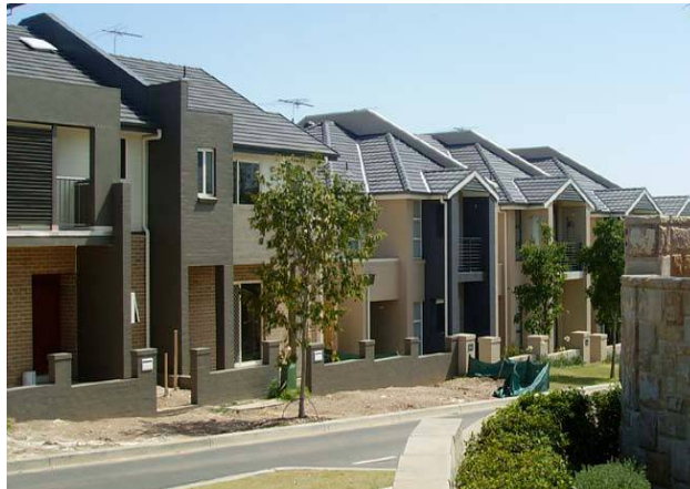
Figure 17 – Broken Wall Planes and Articulation
